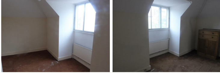
Rear aspect double and secondary glazed window, airing cupboard housing cylinder tank, further storage cupboard.
