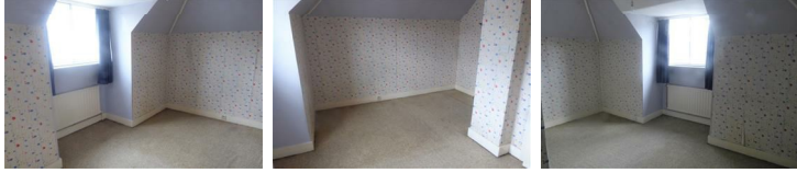
Front aspect double and secondary glazed window, radiator, power point.
